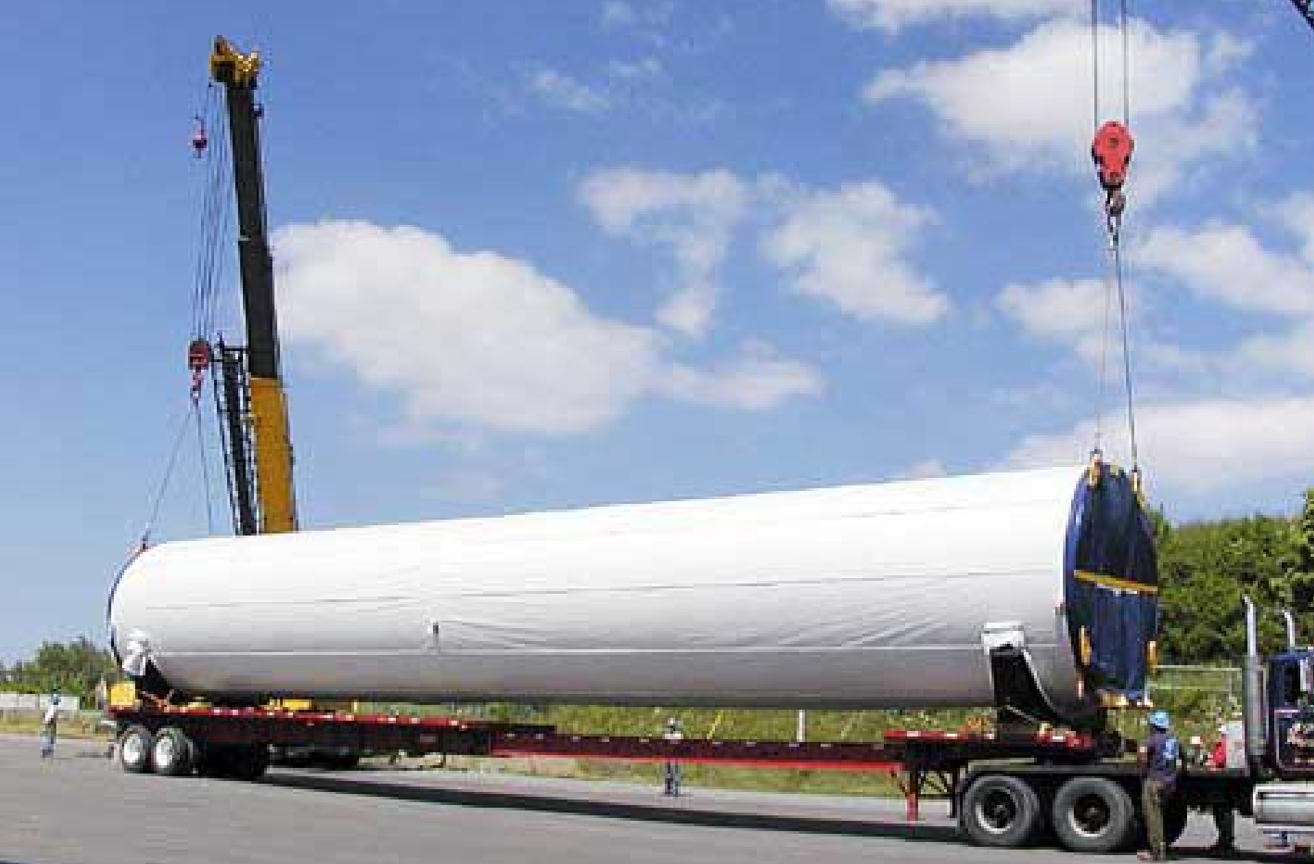
Wind turbine section on truck ready to be transported – 6/21/05
